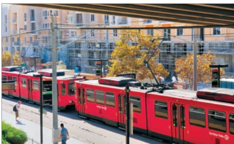
A SANDAG grant helped fund the infrastructure for new development at the Grossmont Trolley Station in La Mesa.
