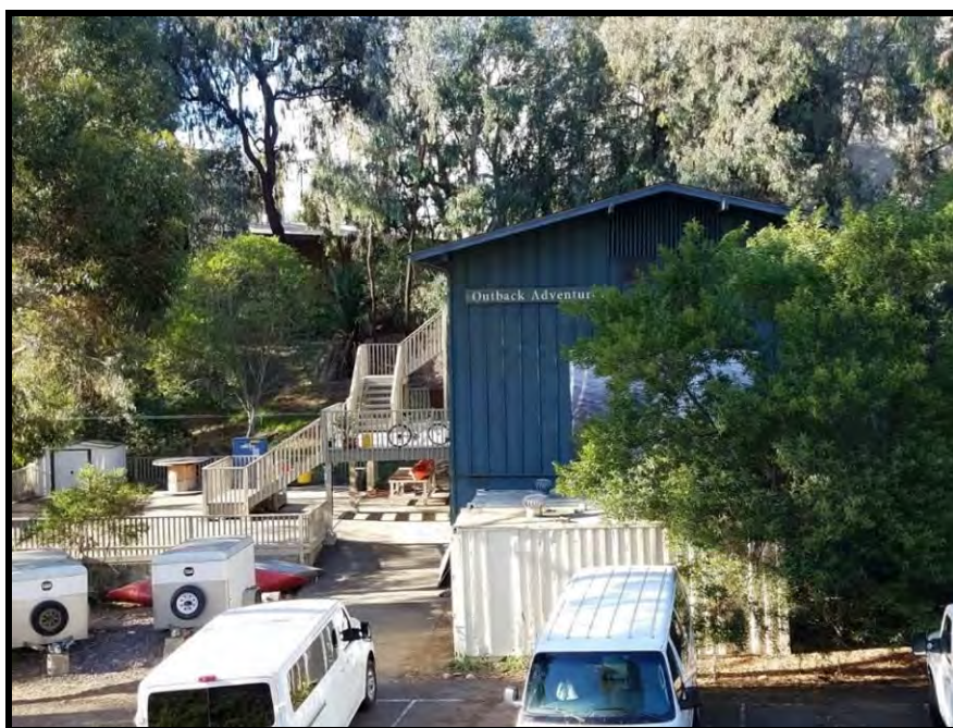
Figure 2-7. Southwestern portion of survey area, Outback Adventures building, view southwest
