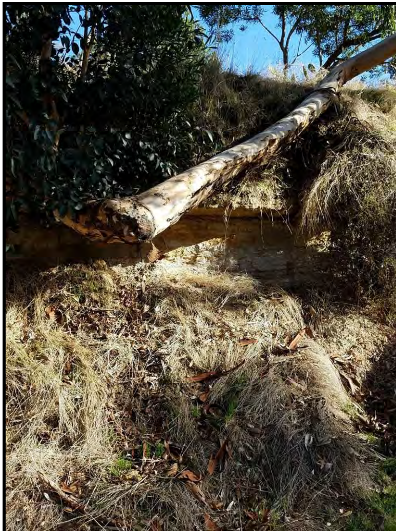
Figure 2-8. Exposed embankment showing likely artificial fill and Scripps Formation, view northeast
