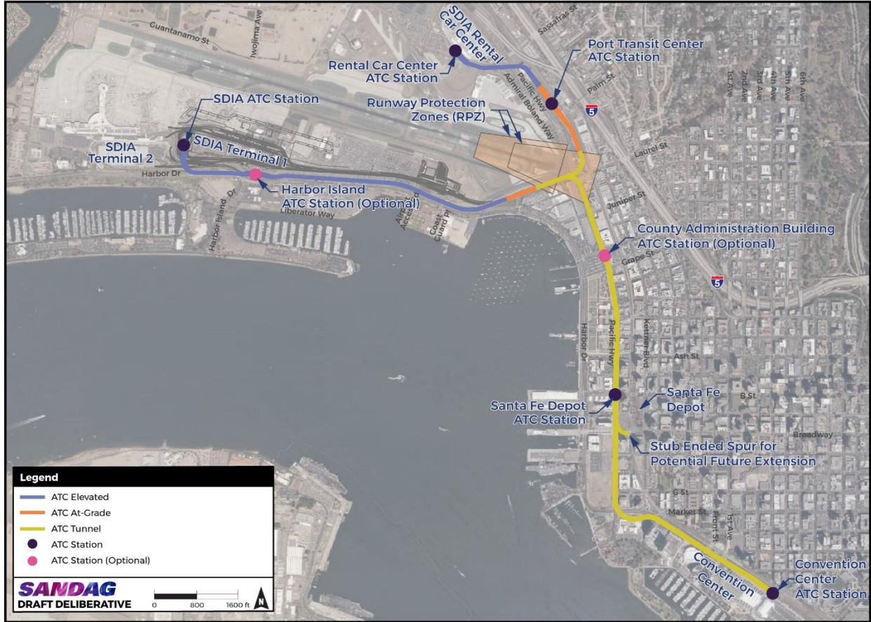
Figure 3-9. Concept 4B Bored Tunnel Airport Transit Connector from San Diego International Airport to Santa Fe Depot Extended to Convention Center
