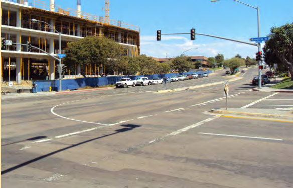
3 Crosswalk striping exists at most intersections, although paint is thinly worn and difficult to see in places.
