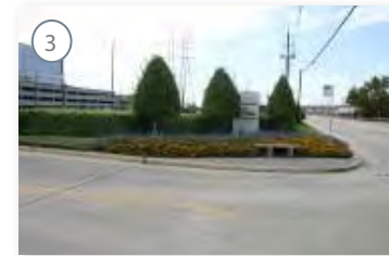
Bad: No landing pad, no ramp, no connecting sidewalk. (Houston, TX). Photo: Christof Spieler
