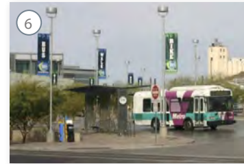
Good: Light fixtures, banners, shelter, paving, and plantings establish pedestrian scale at transit center waiting areas. (Tempe, AZ). Photo: Christof Spieler
