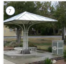
Good: Trash can at stop. (Austin, TX). Photo: Capital Metro
