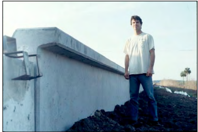
Figure 7. Amphibian and reptile barrier wall at Paynes Prairie State Preserve, along US 441 in Gainesville, Florida © P. Cramer
