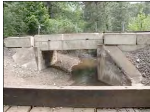
Figure 99. Adjacent culverts and infrastructure just beyond the south side of the interstate (under road & railroad)
