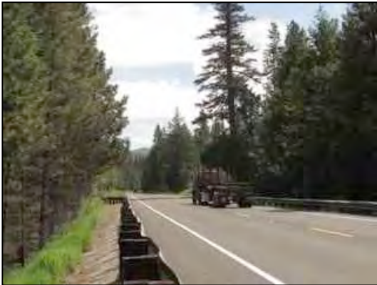
Figure 75. Roadway and adjacent forest
