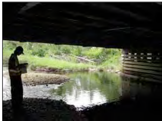
Figure 15. Stream flow through the center span portion of the bridge
