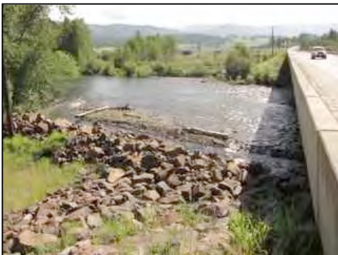
Figure 71. Riprap on east side of river outlet
