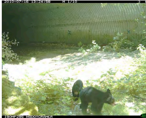
Figure 1300. Black bear cubs following mother through I-90 culvert at mile post 29. Second of two.
