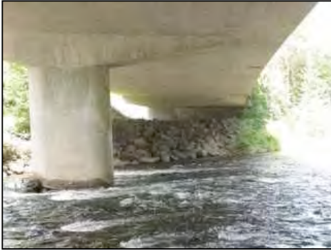
Figure 114. Riprap on west bank
