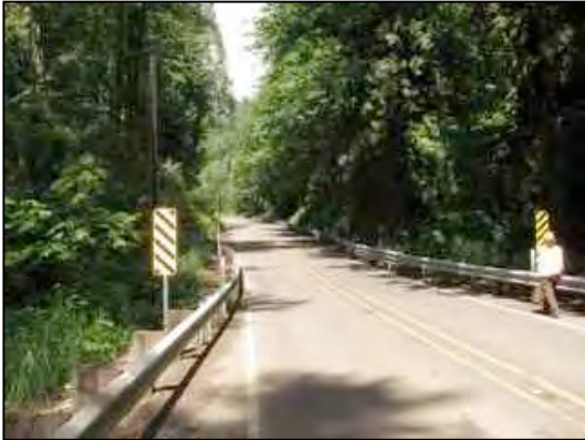
Figure 47. Route 508 looking west
