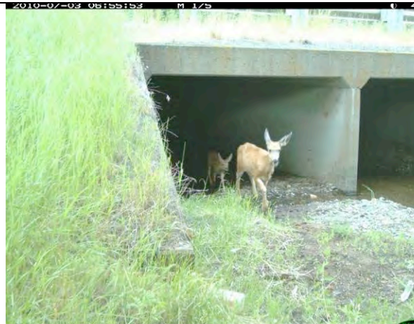
Figure 103. Mule deer brings fawn through the structure under I-90 at MP 73 for the first time.
