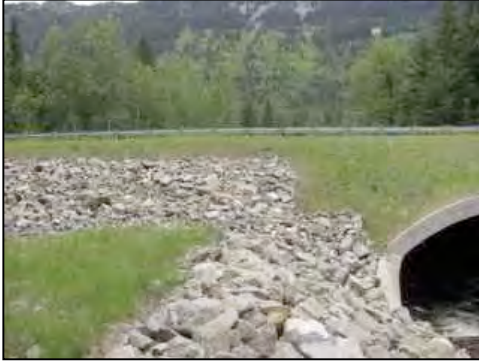
Figure 80. Riprap-lined stream bank and fill slope (north side structure inlet)
