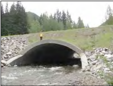
Figure 77. North-side structure outlet
