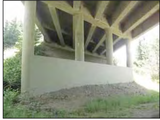
Figure 109. Support wall and side of north structure
