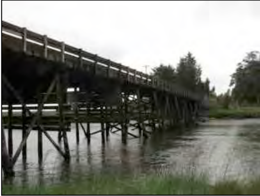
Figure 18 . Inlet side, looking west.
