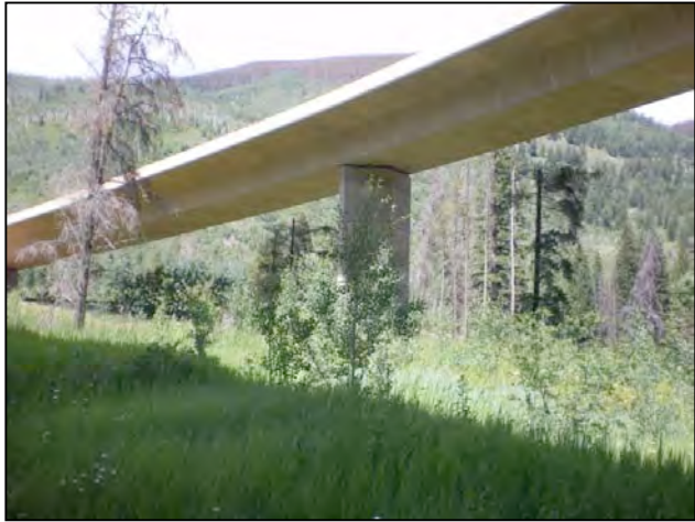
Figure 34. Example of a Class 4 extensive bridge or viaduct, I-70 Colorado © J. Kintsch
