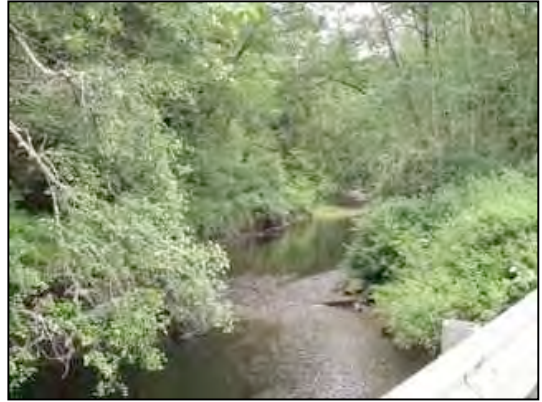
Figure 17. View from structure to east (inlet side)
