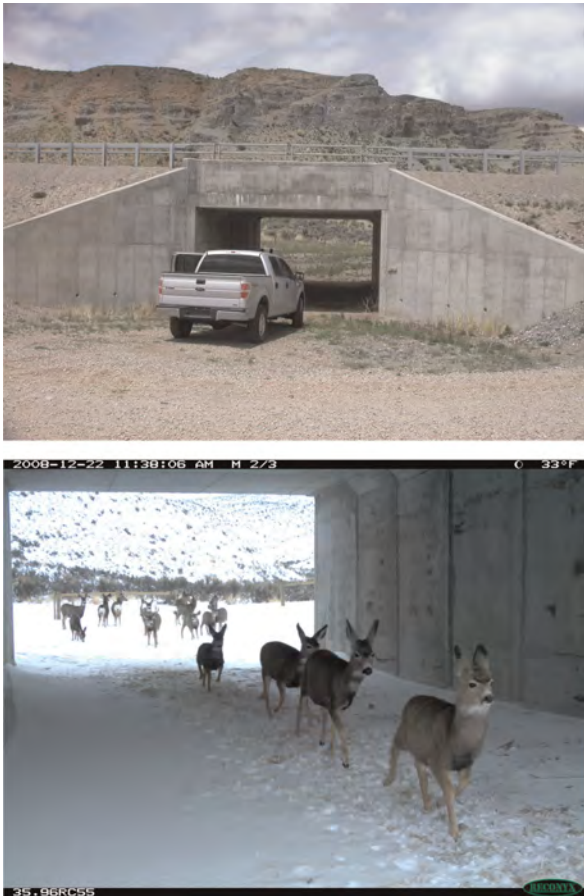
Figure 2. Standard concrete-box underpass along U.S. Highway 30 in Southwest Wyoming, USA, with full-size pickup for reference (top). Mule deer moving through underpass (bottom).
