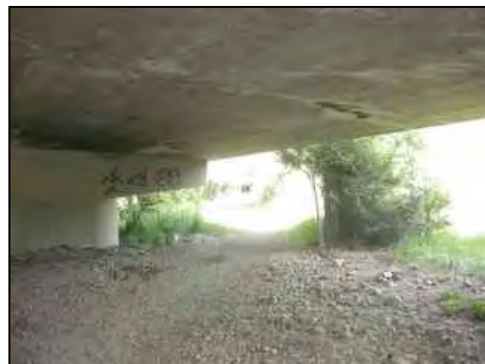
Figure 113. Trail under north structure
