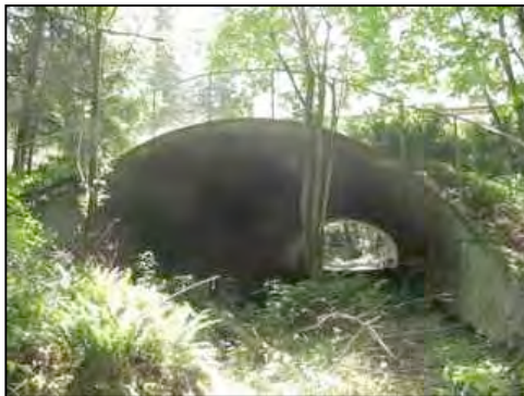
Figure 121. South structure entrance
