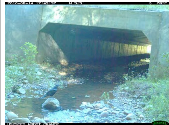
Figure 10. Raven at Mosquito Creek culvert entrance under US 101. There is no evidence the raven went into the culvert.
