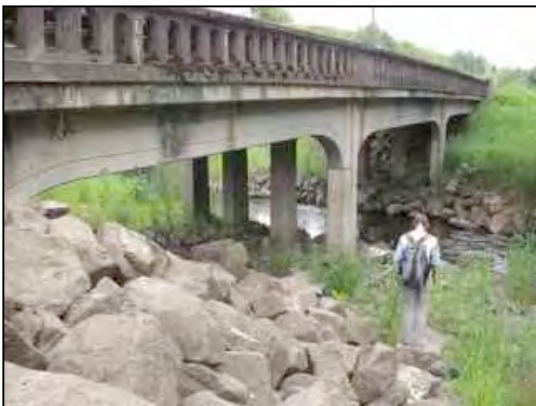
Figure 43. Bridge and riprap side slopes
