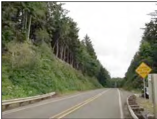
Figure 20 . Roadway looking south
