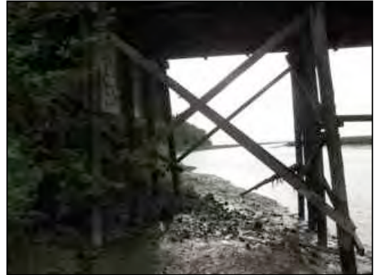
Figure 19 . Bank on south side of structure during low tide.
