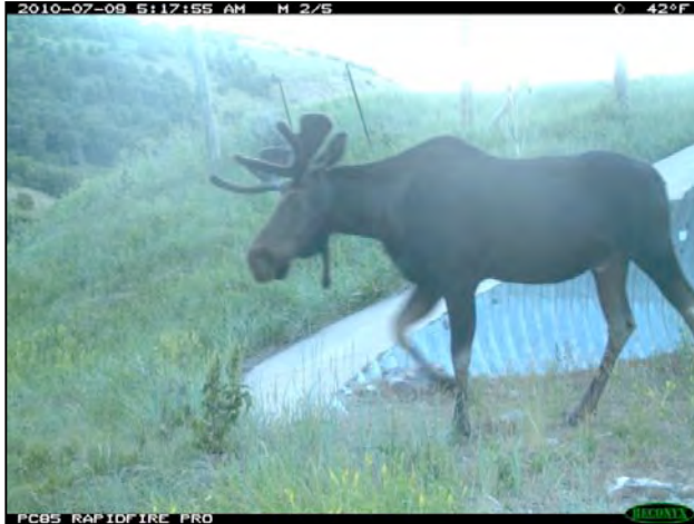
Figure 24. Moose using culvert under US 91 in Utah © P. Cramer
