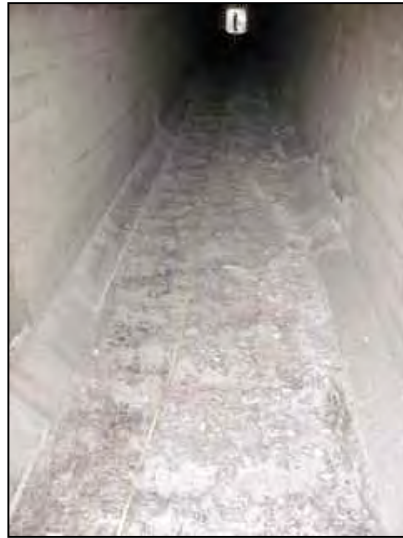
Figure 63. Long, narrow tunnel effect
