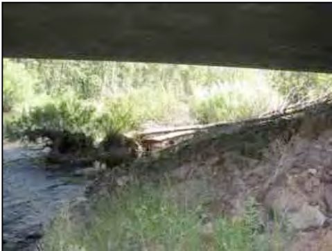
Figure 69. Side slope on west side of river
