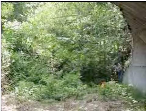
Figure 127. View from north structure outlet
