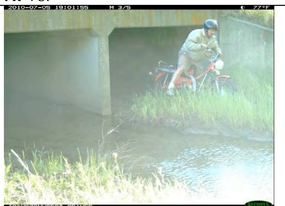
Figure 107. Typical motorized vehicle use of culvert under I-90 at MP 73.
