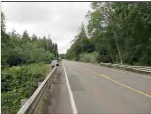
Figure 12. Rte 101 looking North
