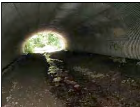
Figure 123. South structure, with unconfined flow
