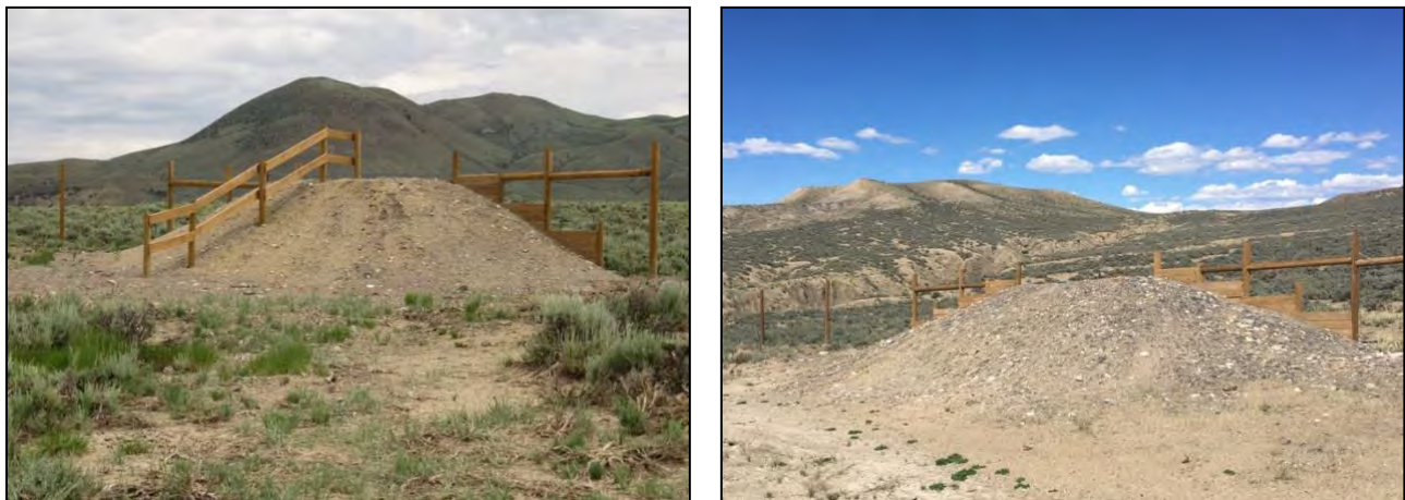
Figure 30. Example of an escape ramp with a 2:1 slope with perpendicular rail fence (left) and a ramp with a 3:1 slope with no rail fence (right).
