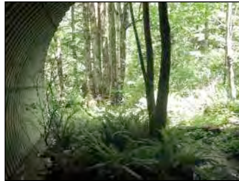
Figure 122. View from structure outlet
