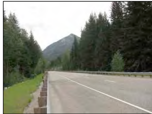
Figure 78. West bound lanes, looking east
