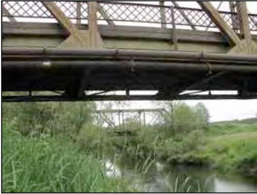
Figure 29. West looking towards bike path bridge
