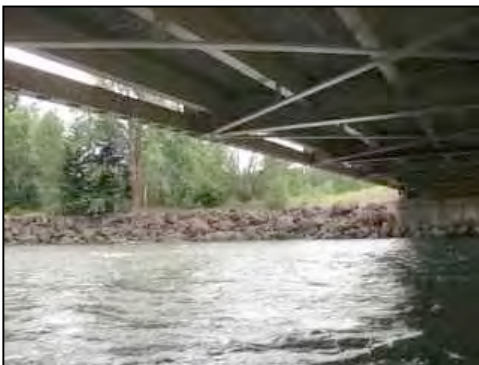
Figure 86. Riprap banks on east side of river
