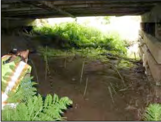
Figure 16. Stream bank under outside span
