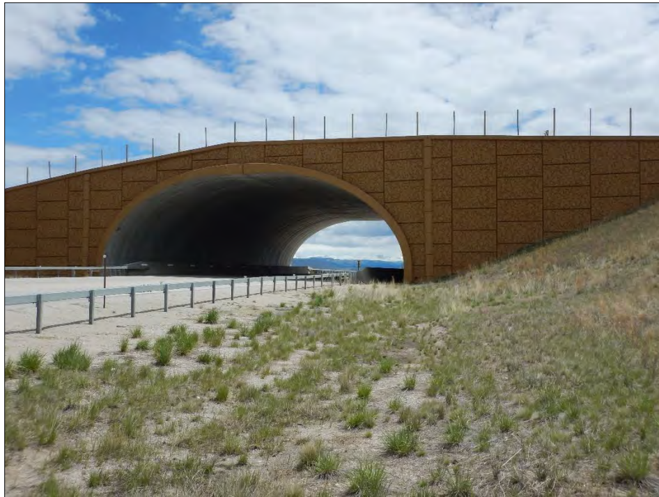
19 Photo: One of the Overpasses at Trapper’s Point with Highway 191 running underneath. 20 21 Credit: Renee Callahan
