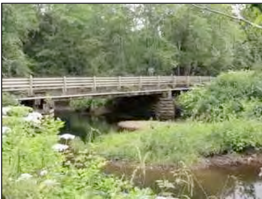
Figure 14. Bridge at Location 101_38.8_02
