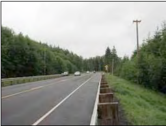
Figure 1. Rte 101 looking south
