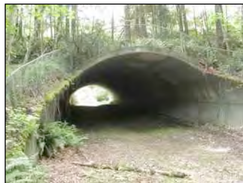
Figure 124. North structure outlet
