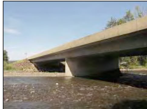
Figure 70. Bridge view from outlet
