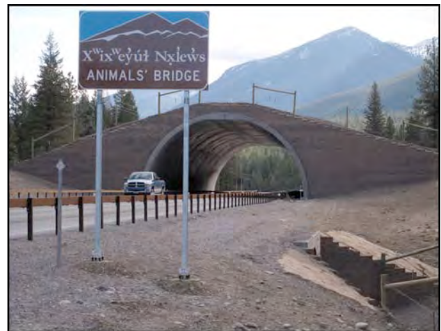
Figure 1. Wildlife overpass over Highway 93, MT © P. Cramer
