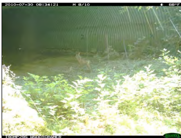
Figure 16. Coyote using culvert under I-90, Washington © P. Cramer, J. Kintsch & WSDOT
