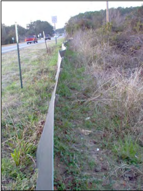
Figure 8. Drift fencing to funnel turtles under the highway to get to other side of Lake Jackson, Tallahassee, FL © P. Cramer
