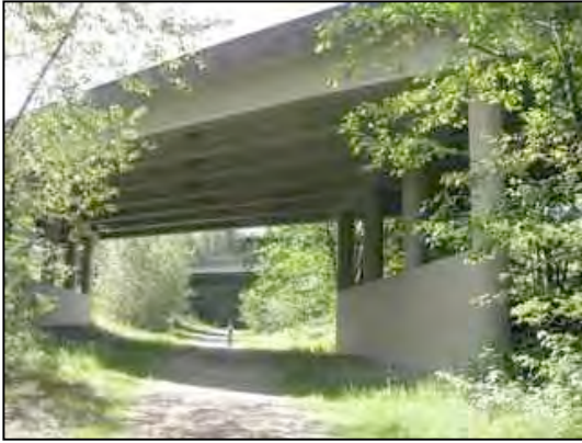
Figure 108. View from north side of slope highway
