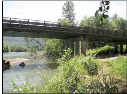
Figure 54. Looking towards inlet
