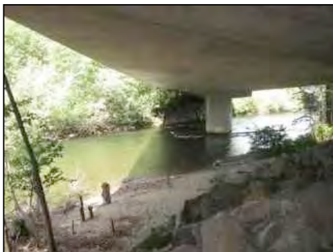
Figure 112. Beneath north structure
