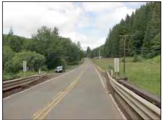
Figure 42. Highway 6 looking west
