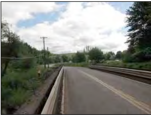
Figure 41. Highway 6 looking east
