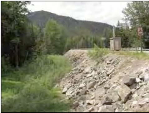
Figure 82. Riprap fill slope on south side (eastbound lanes)
