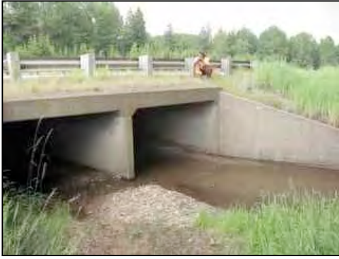
Figure 96. South side outlet
