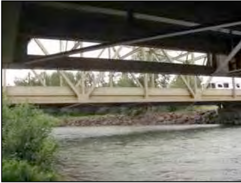
Figure 84. View from beneath south structure
