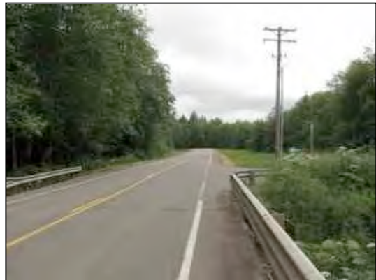
Figure 13. Rte 101 looking South
