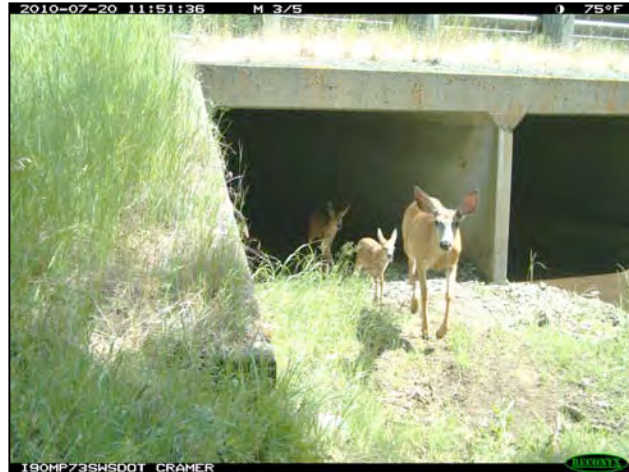
Figure 21. Black-tailed deer doe and fawns crossing under four lanes of I-90 through a pair of double box culverts, Washington © P. Cramer, J. Kintsch & WSDOT
