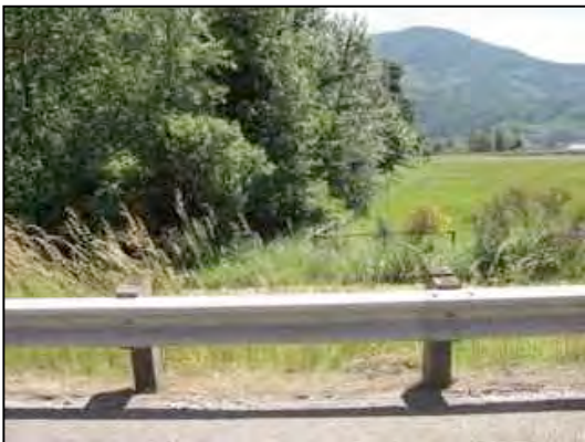
Figure 55. Game trail from riparian Zone and fenced fields to guardrail
