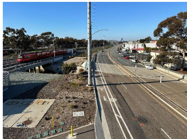
Providing a safe crossing and sidewalk north of the Tecolote Road Trolley Station will make for a more direct connection for people walking from the north.
