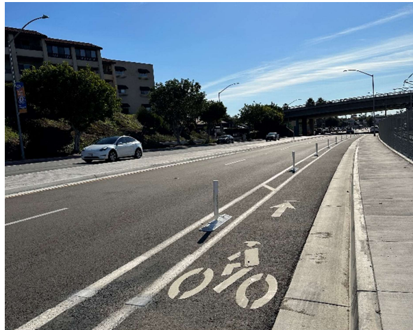
Recently installed southbound cycle track along Morena Boulevard, approaching the Clairemont Drive Station.
