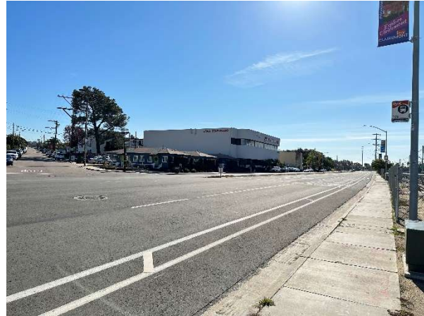
Existing bicycle facilities along Morena Boulevard are currently only provided in the northbound direction and are not suitable with the 40 – 45 miles per hour posted speed limit.
