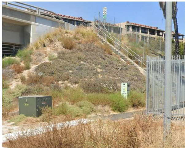
Stairs connecting Clairemont Drive to Morena Boulevard.
