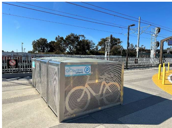
Bike lockers at the Trolley stations provide a secure place to store a bicycle, helping to facilitate multimodal trips.
