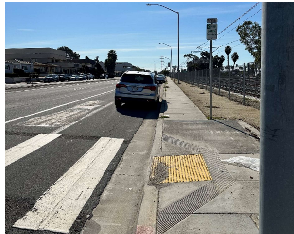
High visibility crosswalk leading to a curb ramp with a detectable warning surface across Morena Boulevard at Ashton Street.
