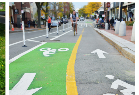
On Street Protected Bike Facility
