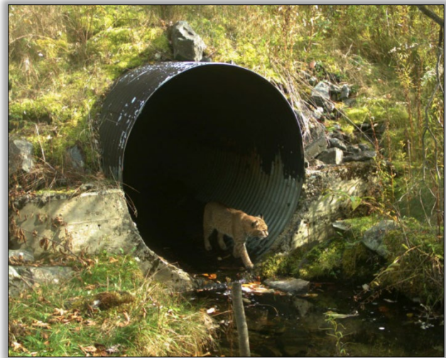
Wildlife Pipe Culvert
