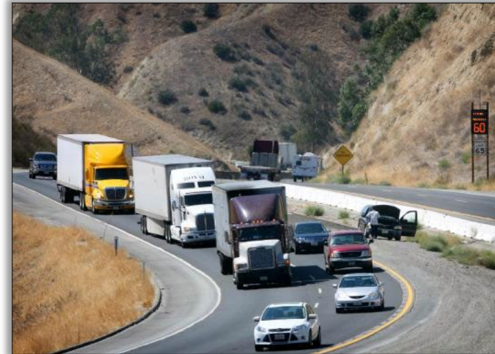
Truck Climbing Lane
