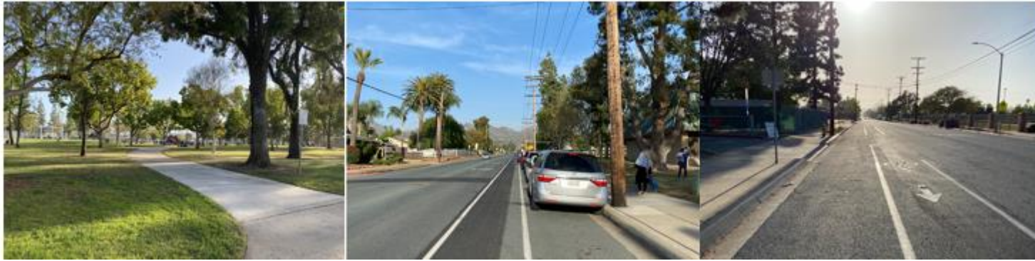
Figure 8. Before Shared Street project implementation in El Cajon
