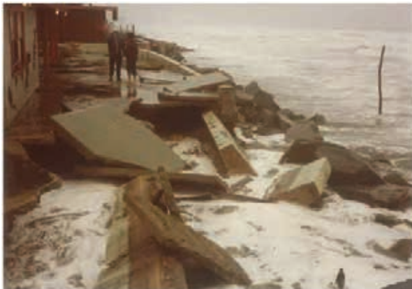
Coastal Damage following 1983 Storm
