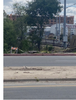
Figure 4. Sidewalk construction on Euclid Ave. near the trolley tracks
