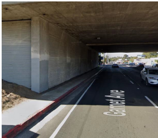
Figure 7: Photo of poorly lit and narrow sidewalk I-5 underpass on Garnet Ave.
