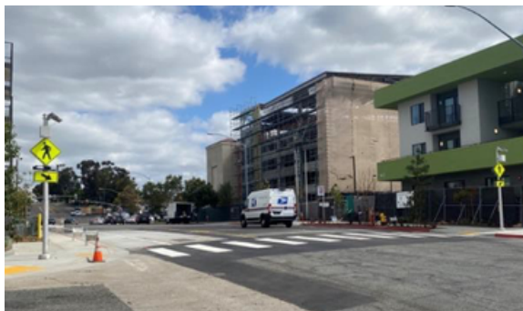
Figure 3: Photo of Hartley & 47th St in Lincoln Park. Well-maintained sidewalk with pedestrian signal and painted crosswalk.
