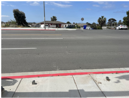
Figure 4. Missing "no pedestrian crossing" sign.
