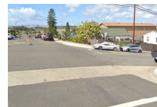
Figure 2. Unlabeled crosswalks at the intersection of S. 40th St. & Gamma St.
