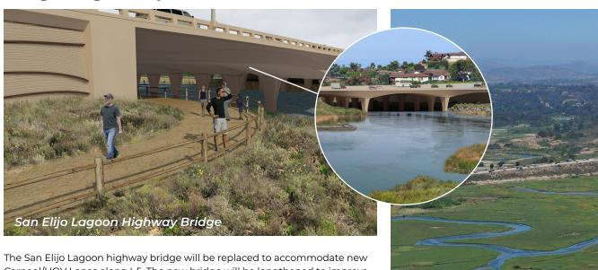
Carpool/HOV Lanes along I-5. The new bridge will be lengthened to improve tidal flows, circulation, and the overall health of the lagoon. In addition, a suspended bike and pedestrian bridge will be built underneath the highway bridge to further increase north-south and east-west connectivity, and create more travel choices. The North Coast Bike Trail will be constructed to expand the regional bike and pedestrian network.
