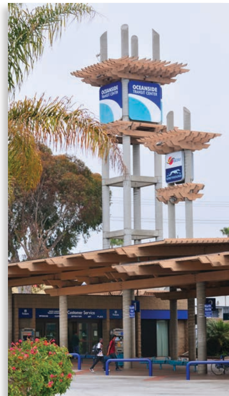
The Oceanside Transit Center serves more than 1.2 million train and bus passengers annually.
