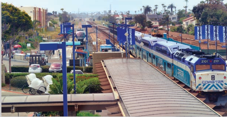
Planned improvements at the transit center include adding a third rail track in the center of the railroad right-of-way, and a 1,000-foot-long boarding platform and passenger walkway at the southern end.
