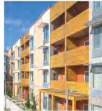
Fig. 3.35 Recessed balconies carved out of the building mass.
