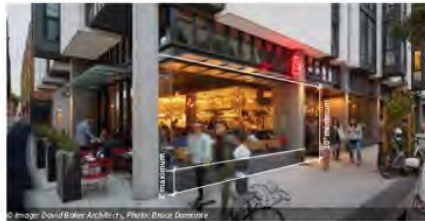
Fig. 4.3 Provide clear glazing for at least 70 percent of active frontage length and have no opaque building elements between 3 to 10 vertical feet of the sidewalk.
